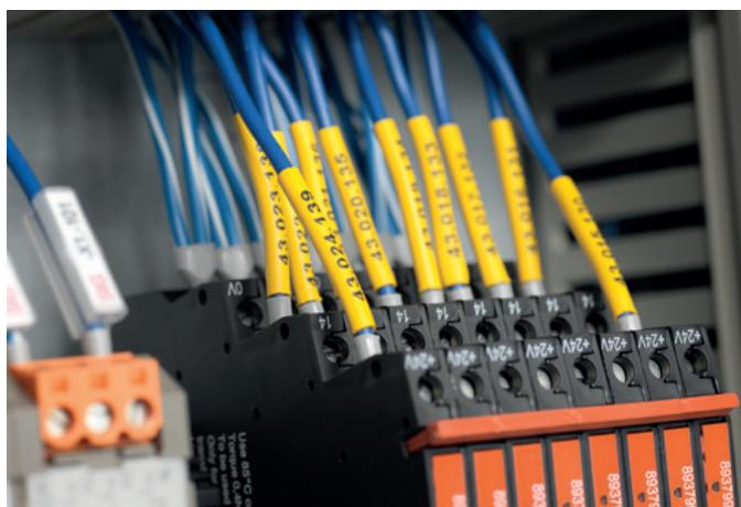
Firm, adjustable seating after shrinking the sleeve onto the wire.
