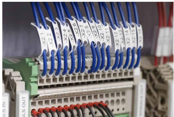
WM markers are available in four sizes for wire cross-sections from 0.25 mm<sup>2</sup> to 16 mm<sup>2</sup>.
