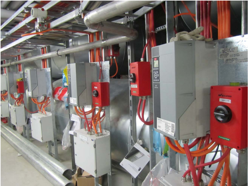
AC drives application with fire rated isolators >
