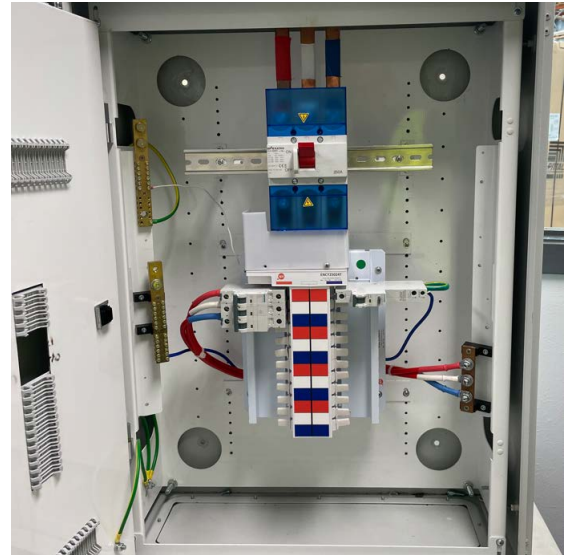
ULTIMATE Distribution Board with EVA3250H main switch
