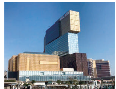
Siemens Energy transformer in MGM hotel in Macau.
